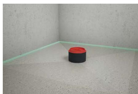
5. Insert floor screed and create a slope to the drain by minimum 2%.
