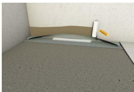
7. Apply liquid waterproofing on both sides of the sealing foil
